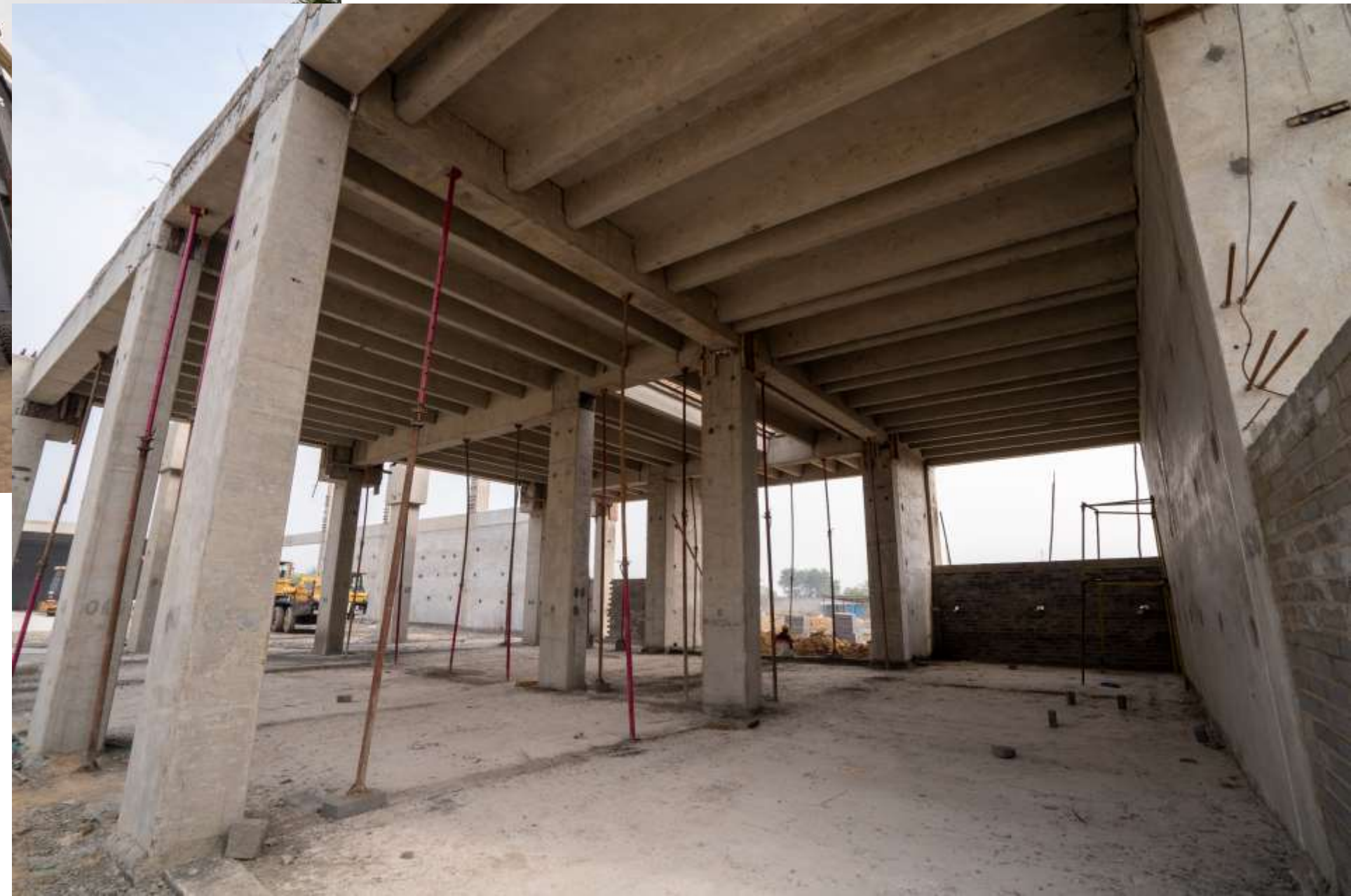
Installed Double T Slab
