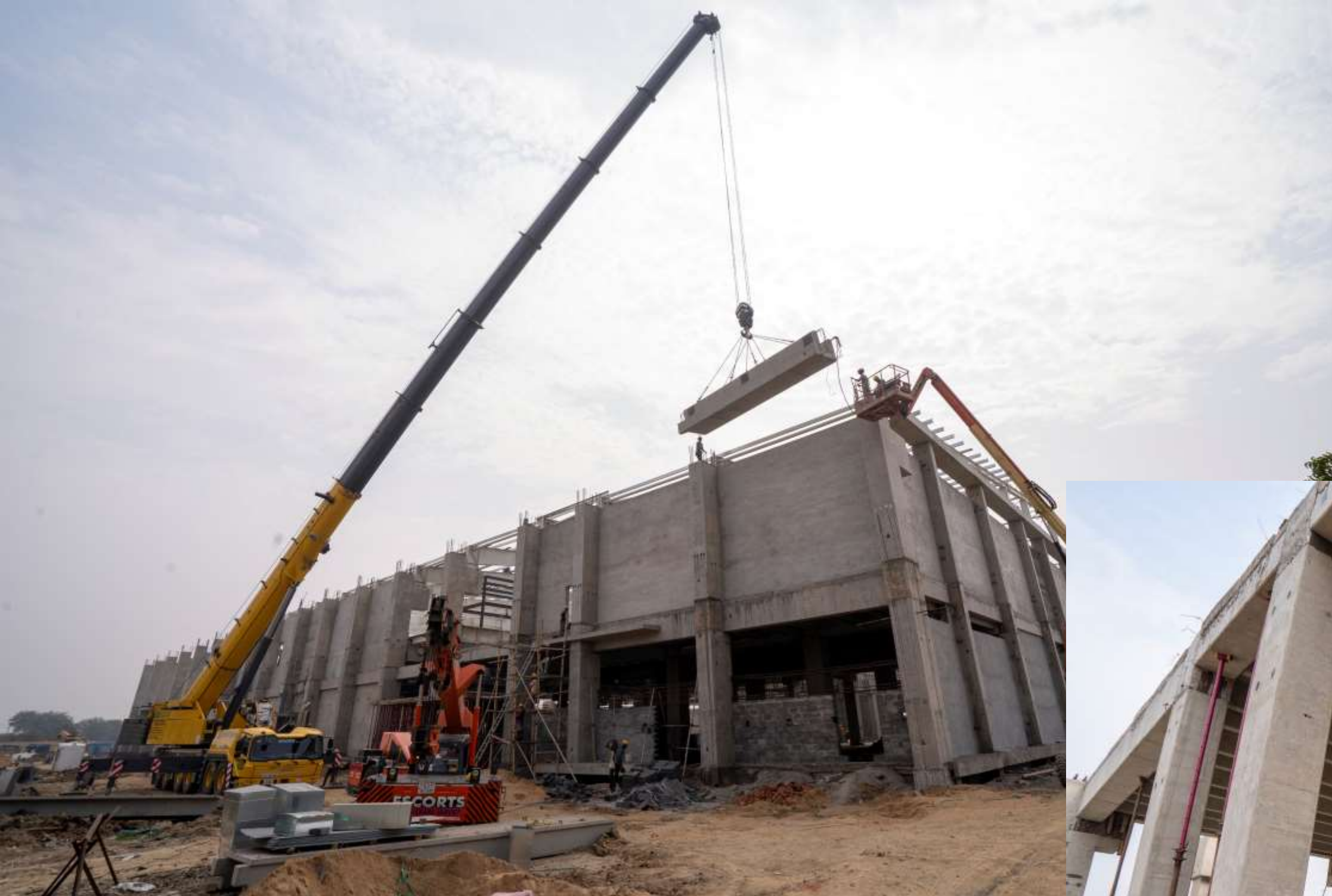
Installation of U-Shape Beam
